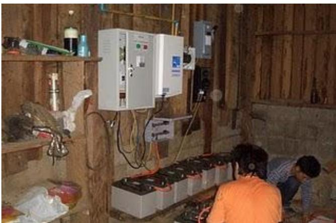
At the first step we installed 14 solar panels, a new charge controller, a new inverter, 12 new sealed solar batteries and a new switch/control unit. The system is build to run also a gasoline generator to charge the batteries if there is not enough sunshine at some days. Because the villagers run a bamboo workshop and us some electric tools which needed a higher amount of electricity so mostly they have to run the generator to cover the daily needs of electricity.
