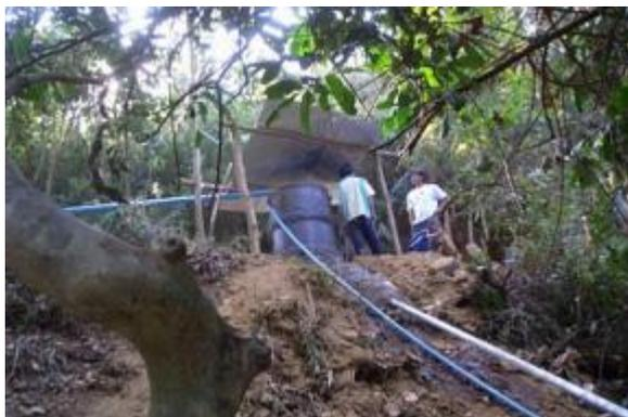
The next well is about 1 km far from the village and because there is no electricity and the long distance we suggest a hydraulic ram pump. The community helps us with the installation and did a great job. After we finished the whole system we increased the water supply to the community tanks and made it possible for them to use their taps like before without walking 1 km down to well to carry water.
