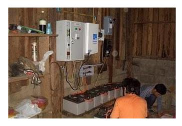
At the first step we installed 14 solar panels, a new charge controller, a new inverter, 12 new sealed solar batteries and a new switch/control unit. The system is build to run also a gasoline generator to charge the batteries if there is not enough sunshine at some days. Because the villagers run a bamboo workshop and us some electric tools which needed a higher amount of electricity so mostly they have to run the generator to cover the daily needs of electricity.
