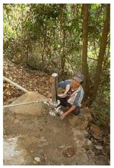
We were able to install a hydraulic ram pump water system around Sop Moey towards the Burmese border. In this village we had to supply water for about 570 people from the Karen hill tribe. They got water through an incline pipe far away but in the dry season the necessary amount of water wasn't sufficient enough.
