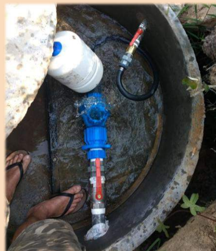
Installation of Ram Pumps
